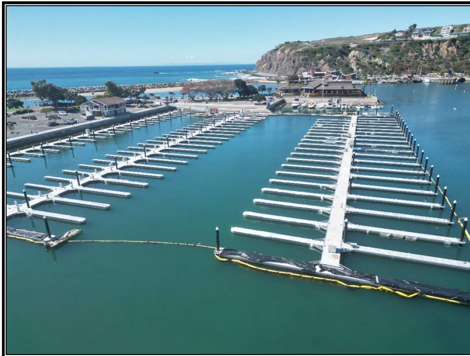
PHOTO 6: View of docks in construction phase (Phase 8), West Island area.
