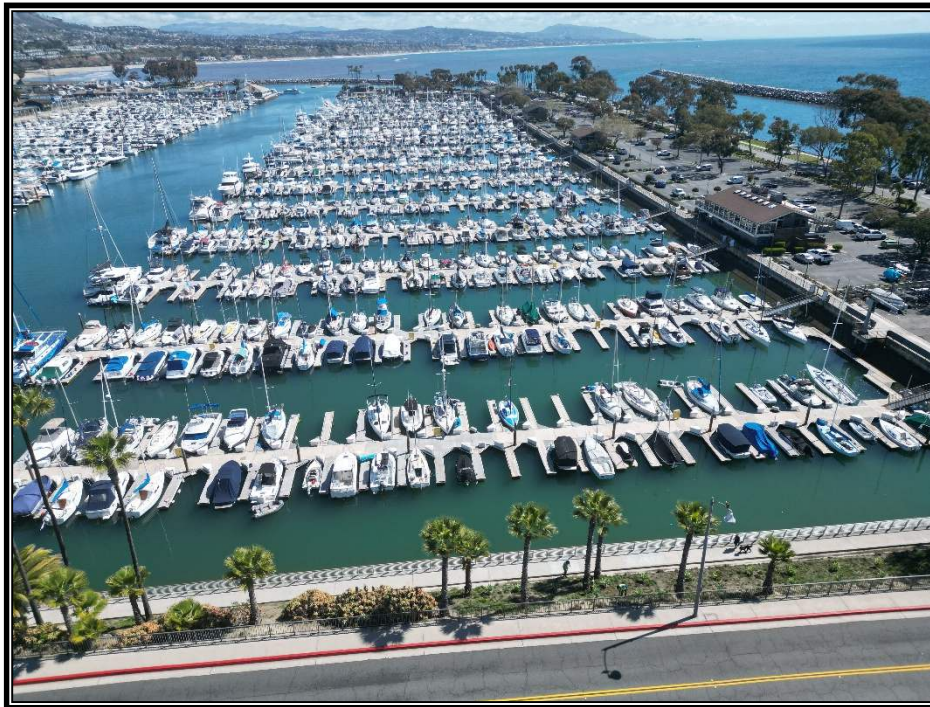
PHOTO 4: View looking easterly at East Island area.
