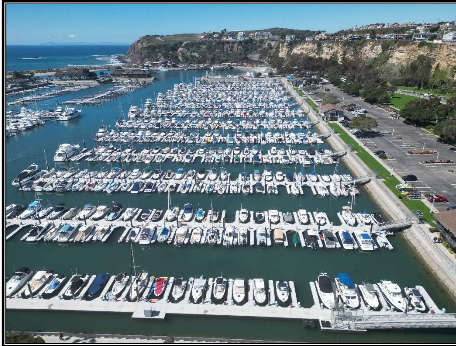
PHOTO 1: View looking westerly at West Cove area.
