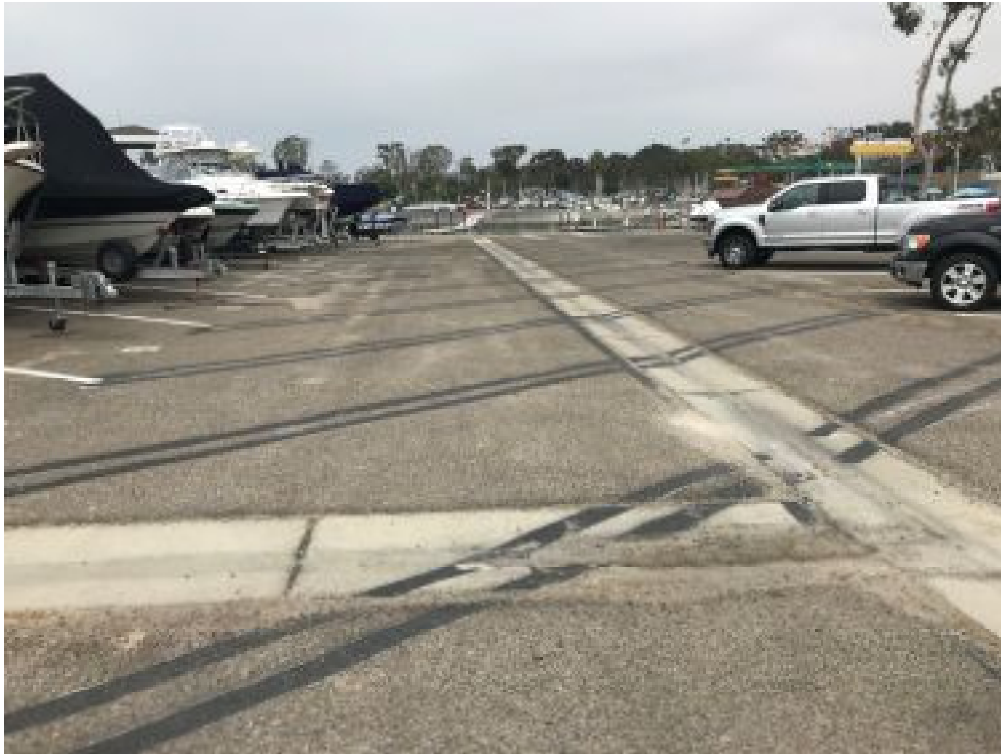
Outlet 2 (6-inch orifice)
