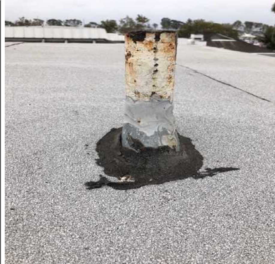
33. Roof above the Killer Dana store. ACMB roof mastic.
