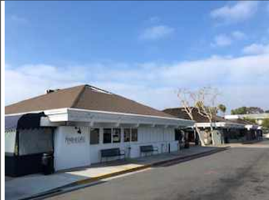
7. Exterior view looking West toward Harbor Café Restaurant.
