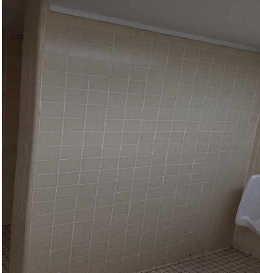
39. 34571 Golden Lantern. Lead-based Beige Ceramic Wall Tile in Men's Restroom.
