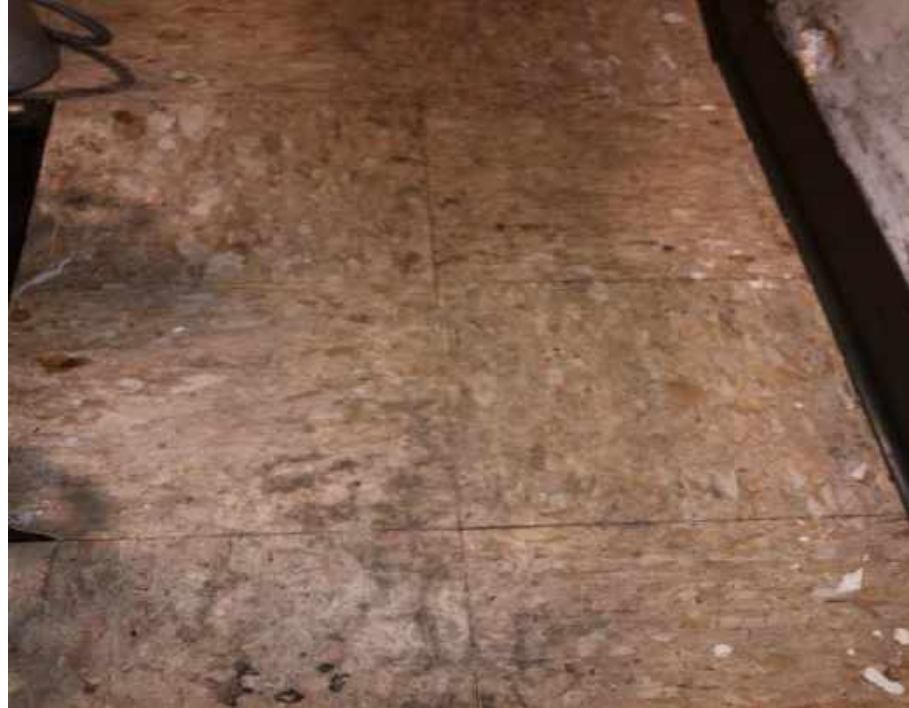
27. Wind & Sea Restaurant. ACBM 12" vinyl floor tile.
