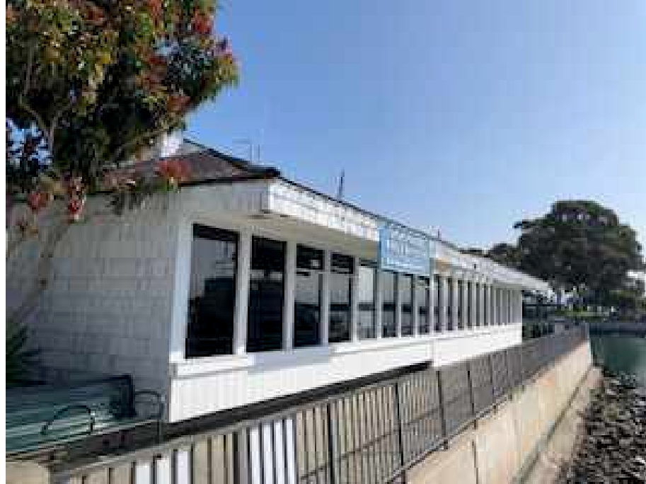
13. Exterior view of the Dana Wharf Sportfishing building.
