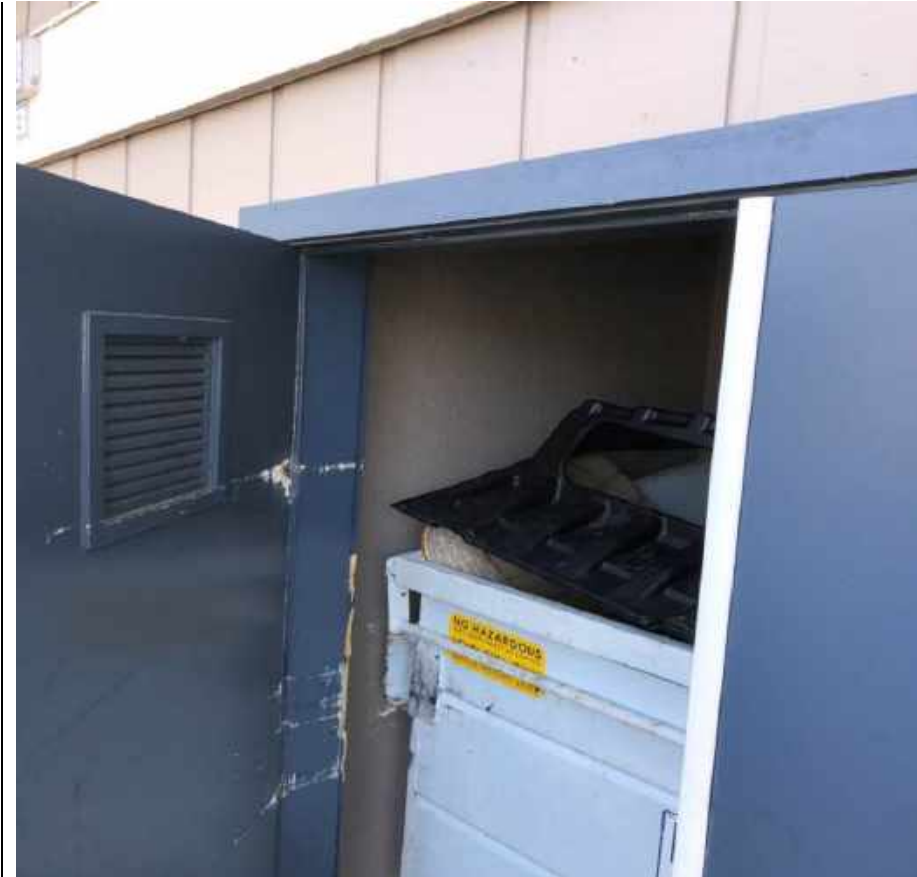
35. 2nd Boater's Building ACCM exterior stucco.
