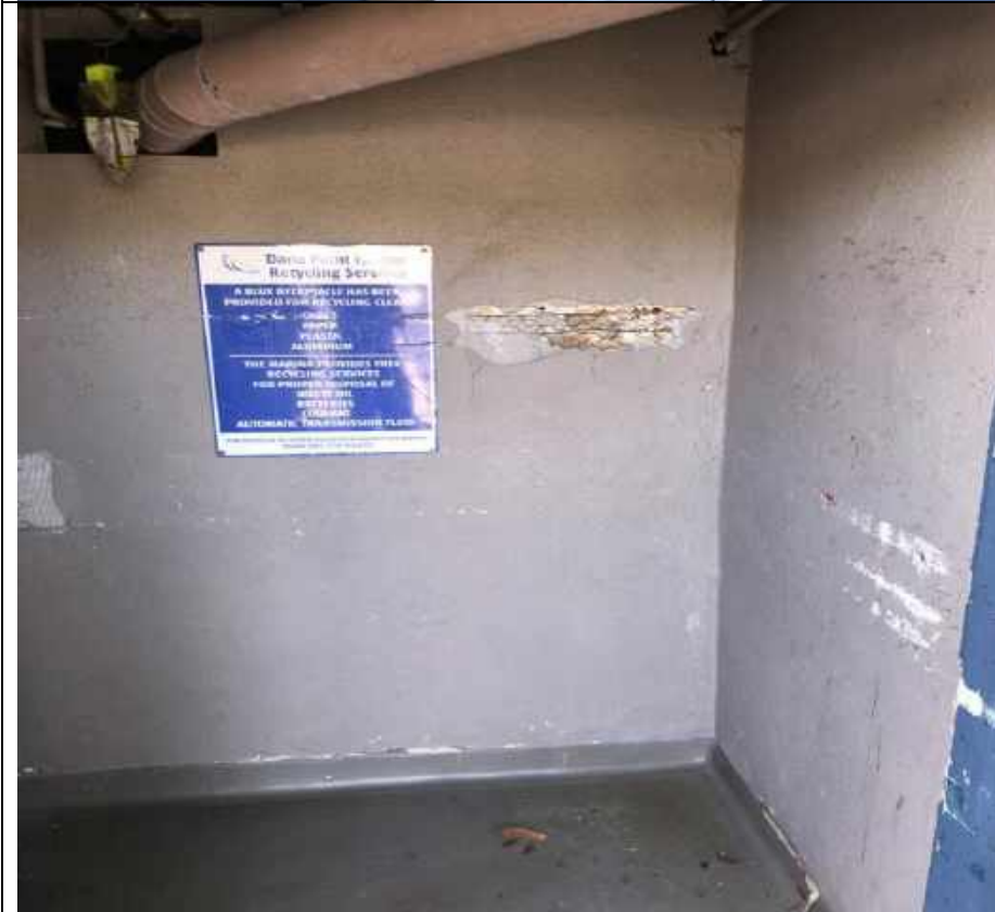
36. BWP Management Building. ACCM exterior stucco.
