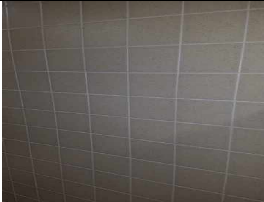
40. 34571 Golden Lantern. Lead-based beige ceramic wall tile in Men's restroom.
