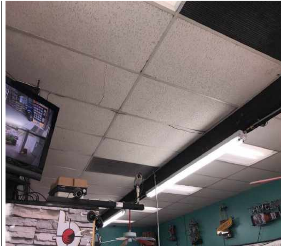
23. Village Market ACBM acoustic ceiling panels.
