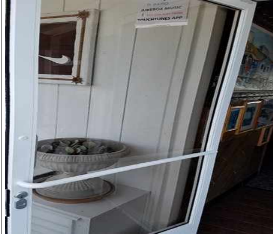
53. Turk's Restaurant Lead-based painted white metal door.
